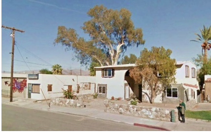
Existing Buildings. SOURCE: Michael Baker International
