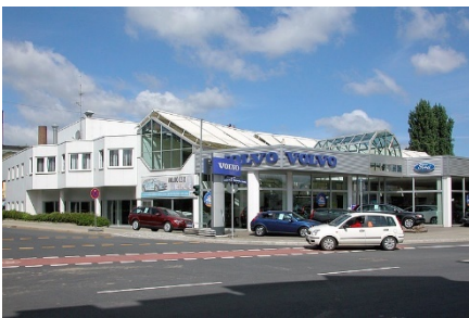
Examples of Pedestrian Friendly Automobile Oriented Commercial/ Light Industrial Buildings. SOURCE: Michael Baker International
