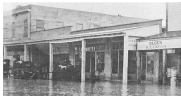
Classic Old West Architecture (Use of Colonnade)
