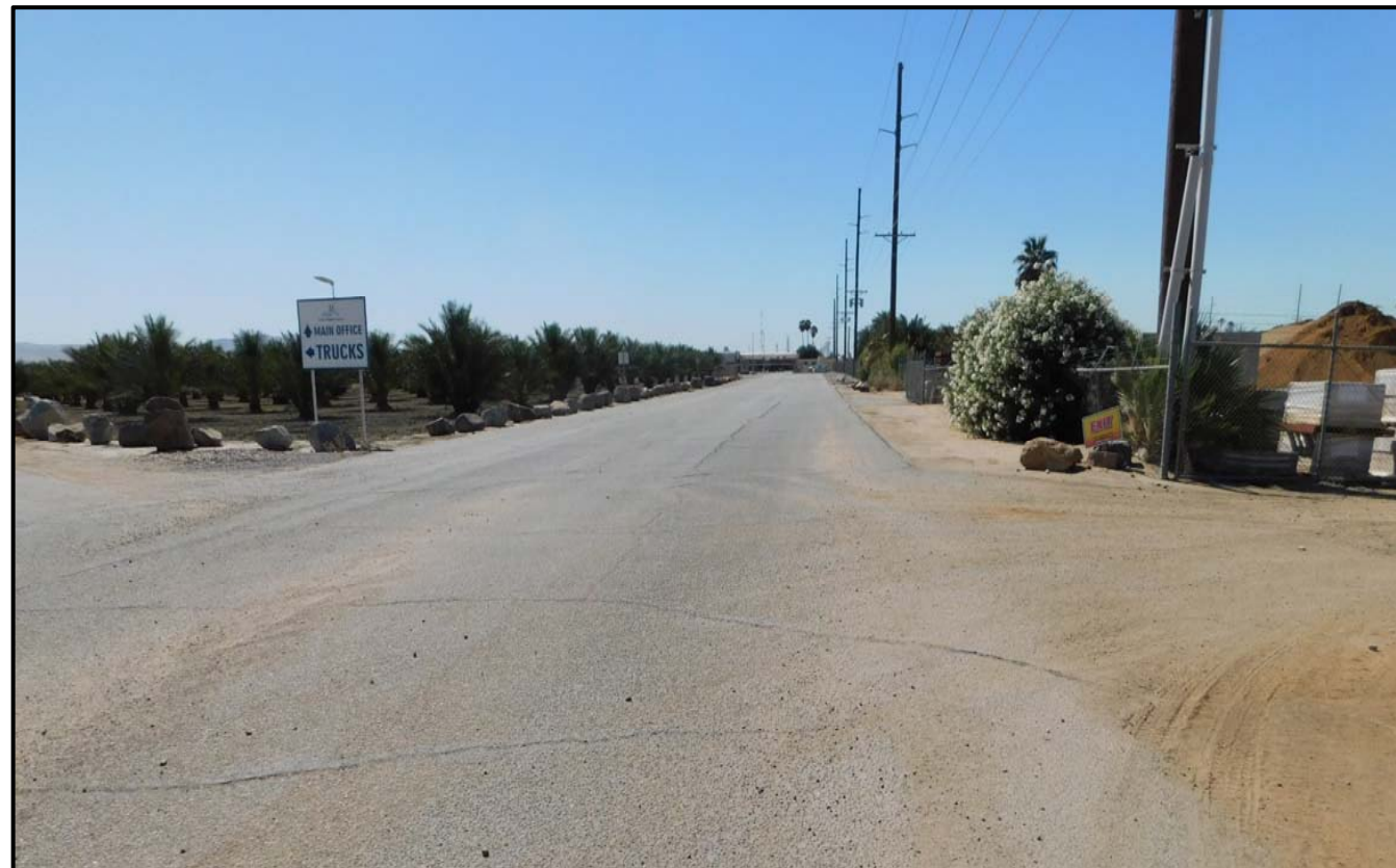
View from Northwest Corner of Site Looking Southeast
